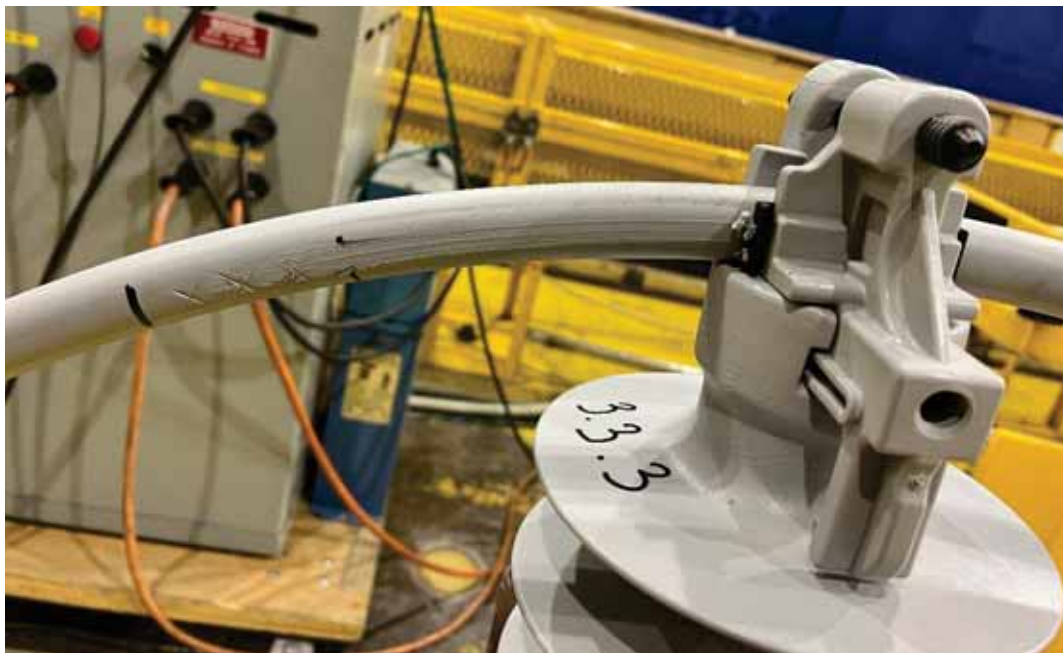
Figure 6-20: Sample 3.3.3 - 22 kV, 397.5 kcmil AAC Condition after Test
