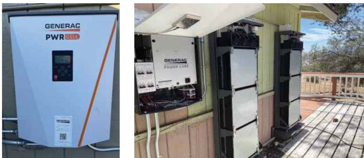
Figure 8-6: FPB Installation at Mobile Home Park Community
