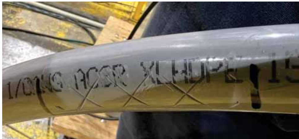
Figure 6-15: Sample 3.2.2 - 35 kV, 1/0 AWG ACSR Condition after Test
