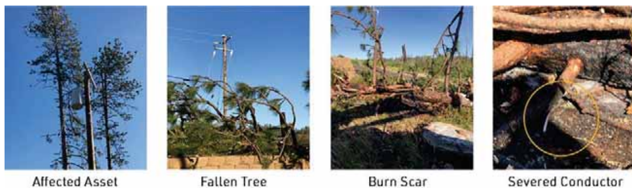
Figure 2: PG&E Covered Conductor Effectiveness – Example 1
